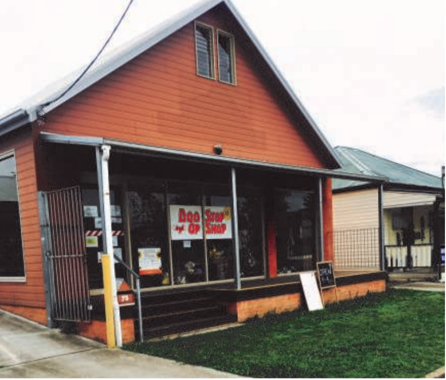
■ The new Doo Stop Op Shop at 75 Maitland Road, Branxton has been opened to help fund a local domestic violence refuge Jodie's House at North Rothbury
