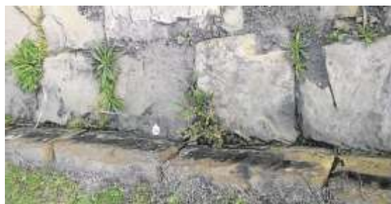
• Sandstone Kerb & guttering in Drinan St, Branxton
