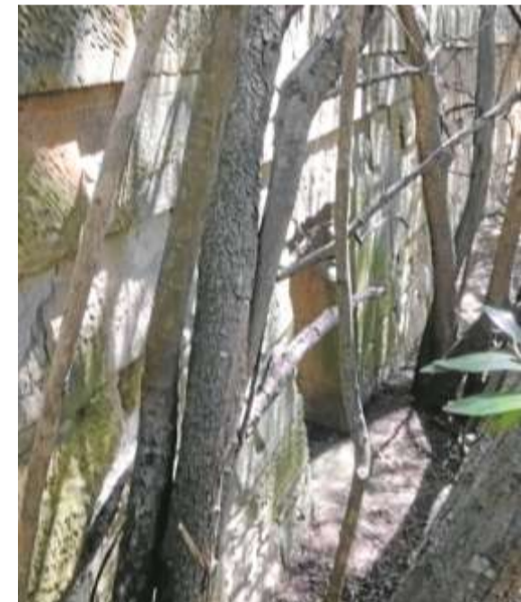
• The wall that holds the convict tunnel
