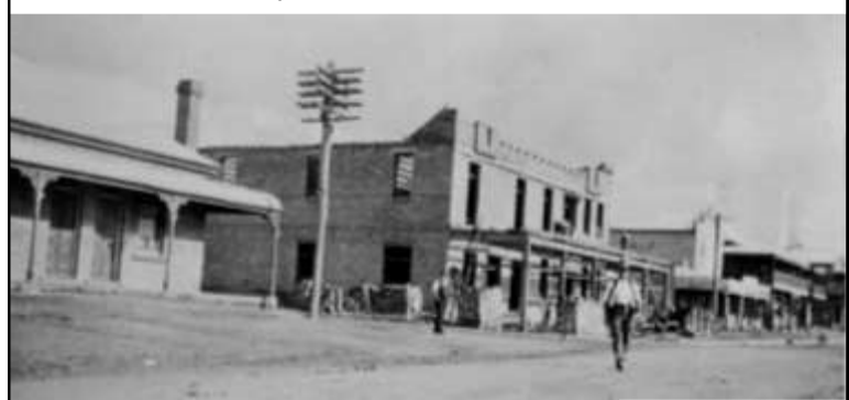
■ Above: The Royal Federal Hotel Branxton under construction
