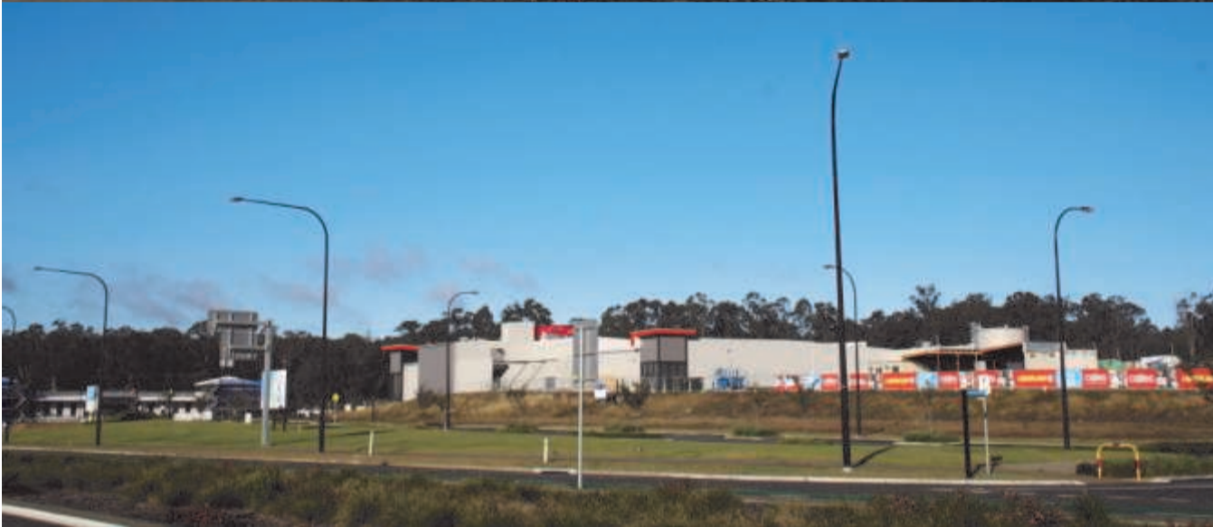
☞ Above: The new Coles complex at Huntlee almost complete
