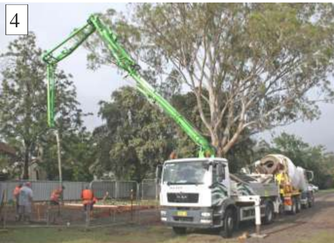
■ Concrete pumper at work
