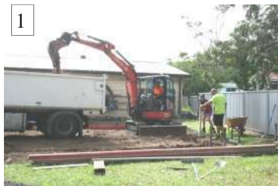
■ Excavating the foundations
