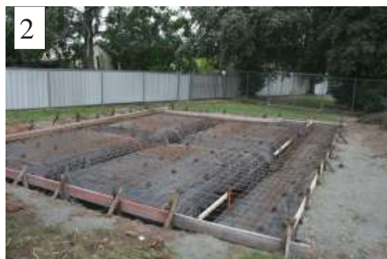
■ Foundations formed and ready for concrete
