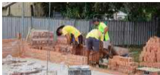
To early days bricklaying ....
