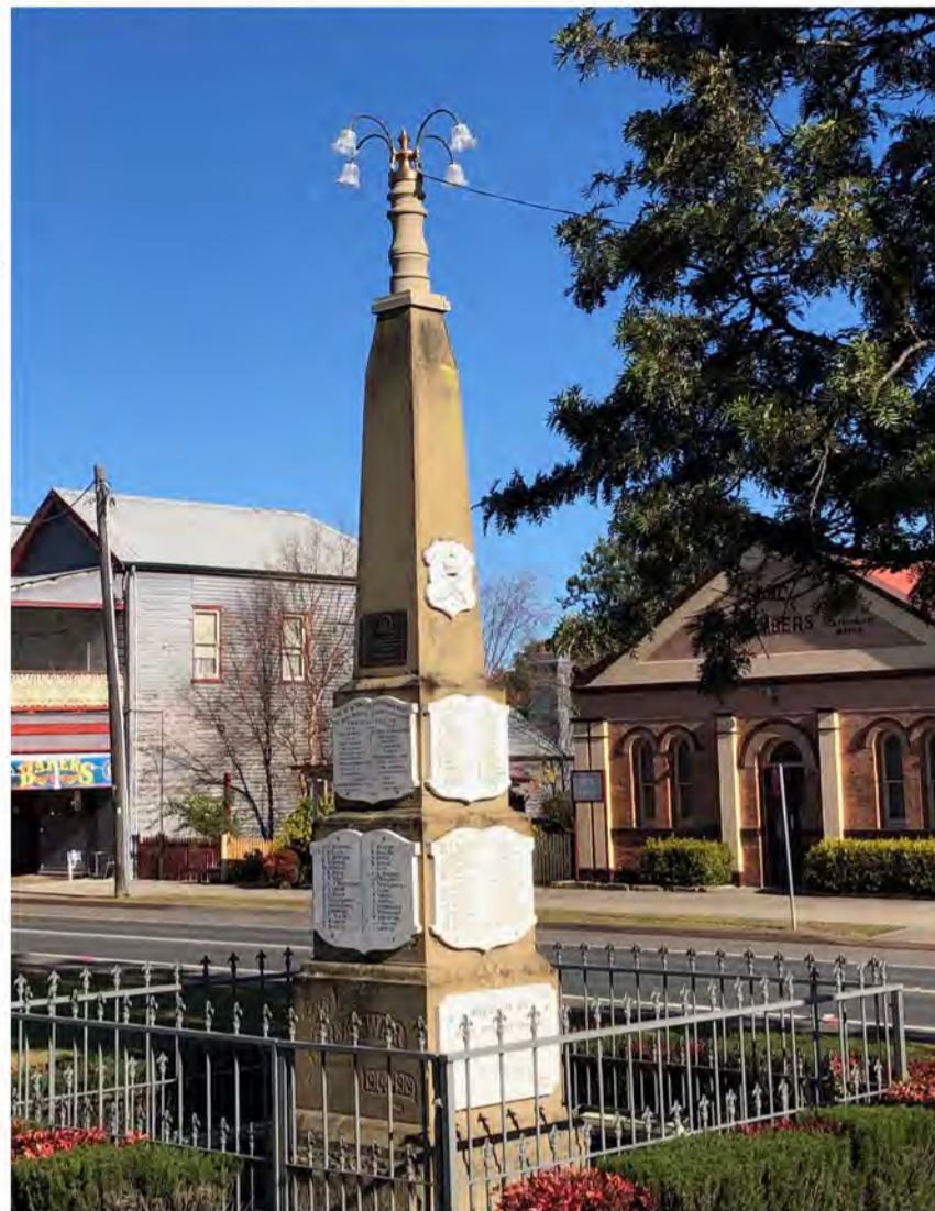
# The new sandstone top and lighting which was put in-situ last week & ready for its official recognition
